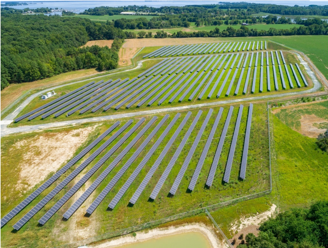
Example of single-axis tracker solar farm
