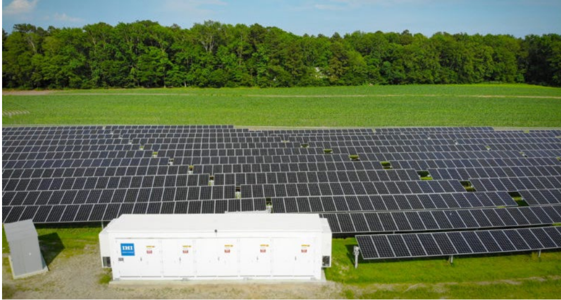
Example of a BESS. Source: IHI Energy Storage
